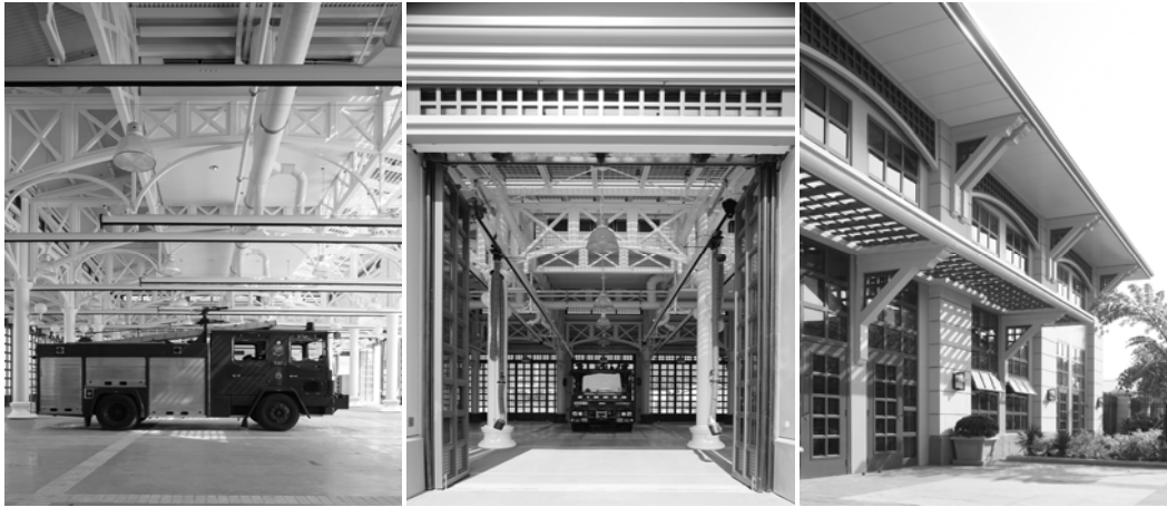
Figure 5: Penny's Bay Fire Station
